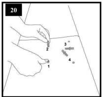
Position and push in the 4 rawplugs. These must be flush with the coping.
